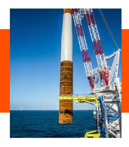
While HaloCAM has initially been developed for subsea applications, the sensor (in slightly different physical form) can also be used on the surface for structure pile/WTG monopile installation.
